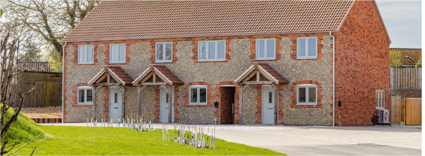
Completed terrace, Norfolk flint and brick with oak-framed porches
